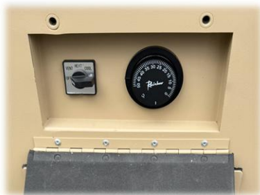
Unit Mounted Controls
